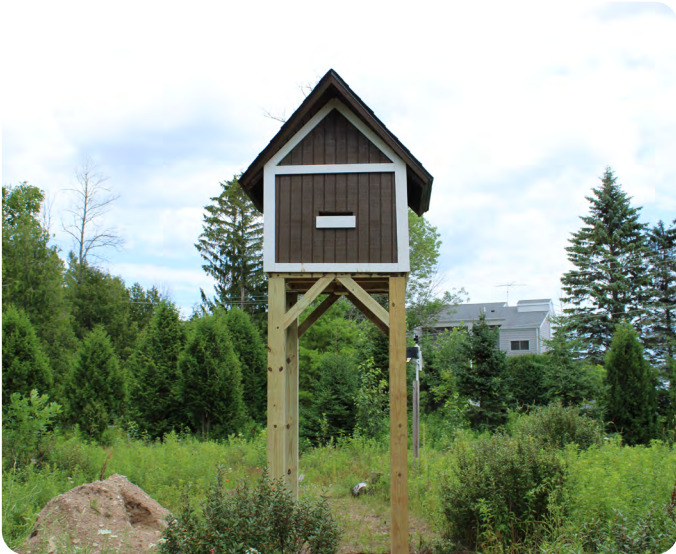
Newly installed bat houses help protect these sensitive species
