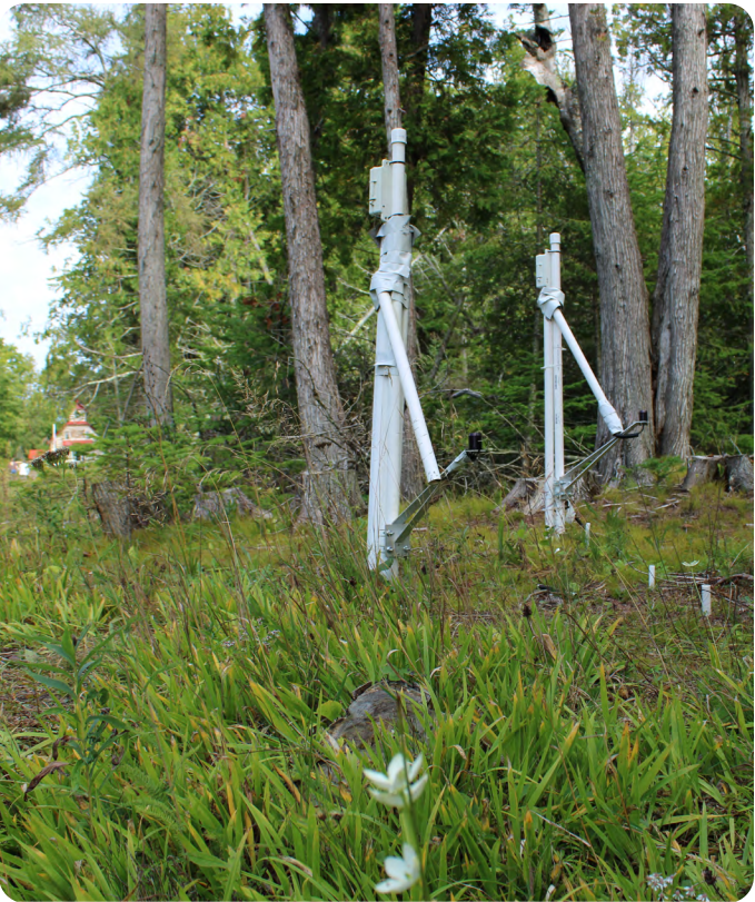
Hobo monitors at the junction of the Range Light Corridor and Wintergreen Trail
