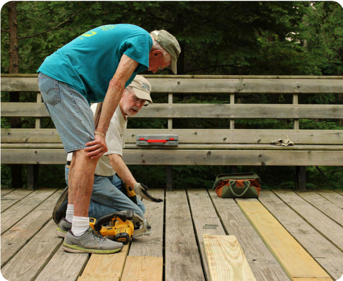
Wednesday Crew volunteers replace boards on swale overlook
