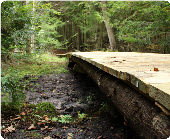
A new boardwalk segment protects sensitive soil from foot traffic at Logan Creek
