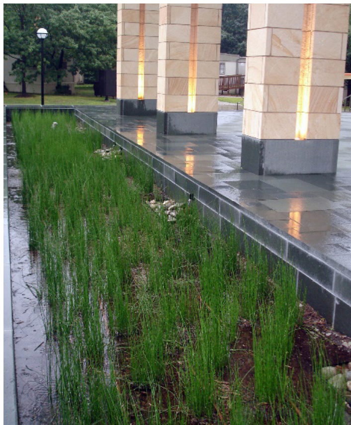
Figure B41: Bioswales treat runoff from hardscape surfaces.
