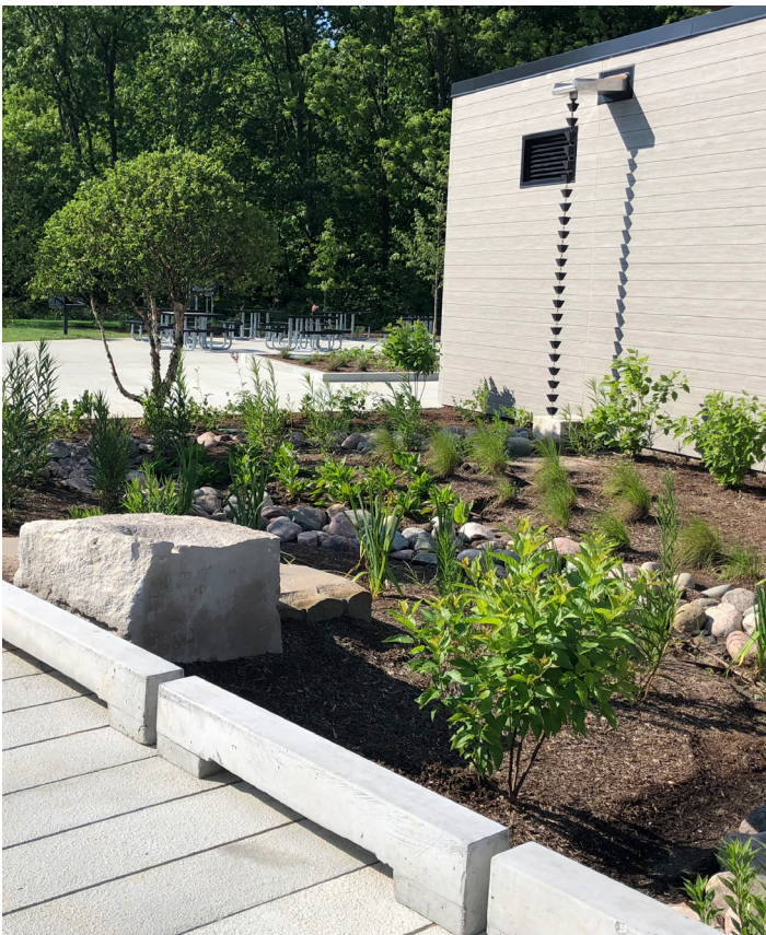
Figure B39: A rain chain directs roof runoff to a bioswale for treatment.
