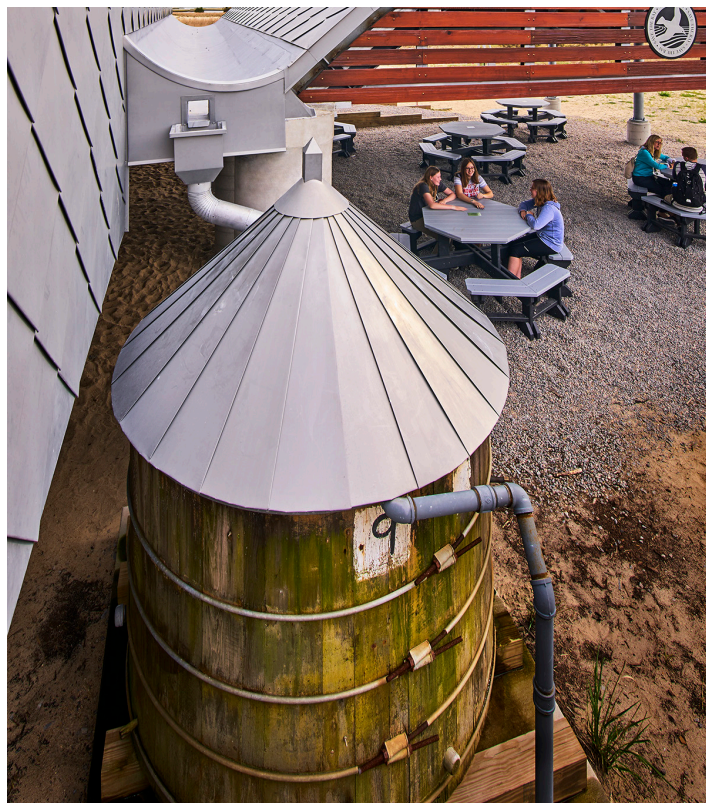
Figure B40: Cisterns can be used to collect roof water to meet non-potable water needs.
